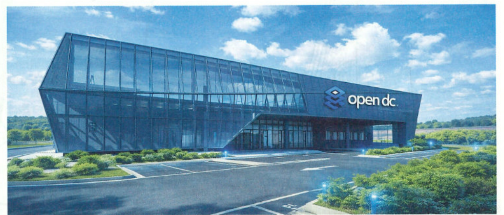
Open DC's data centre facility will house an internet exchange
